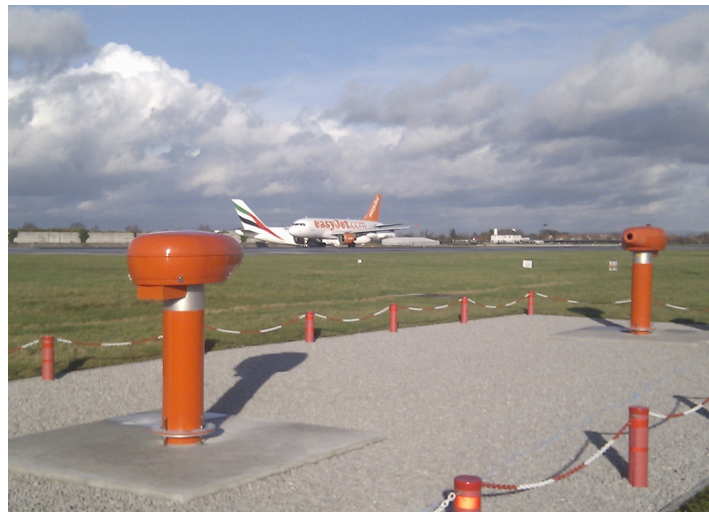
Figure 4: Transmissometer Installation
